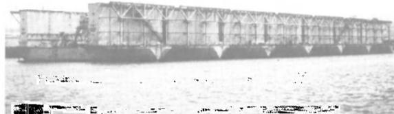
The seven-section floating drydock berthed at Pearl Harbor, Hawaii, will be transported to the new Sabine Yard of Bethlehem Steel Corporation on Pleasure Island. The seven-section, open-ended unit has a lifting capacity of 56,000 tons. It is one of the largest floating drydocks in the country.
