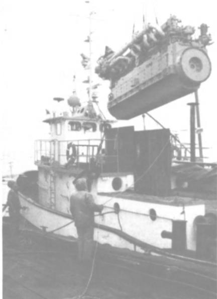
The Stork-Werkspoor 9FHD-240 diesel engine being lowered into the Brenda H.
