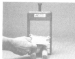
Install stay plate above first row. Install additional rows of cables and stay plates as required.
