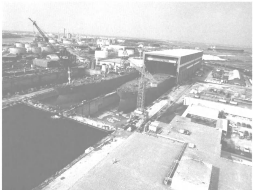
The erection & assembly building—600' x 145' x 115' with three-250 ton bridge cranes—spans 350' of Dry Dock No. 4.
