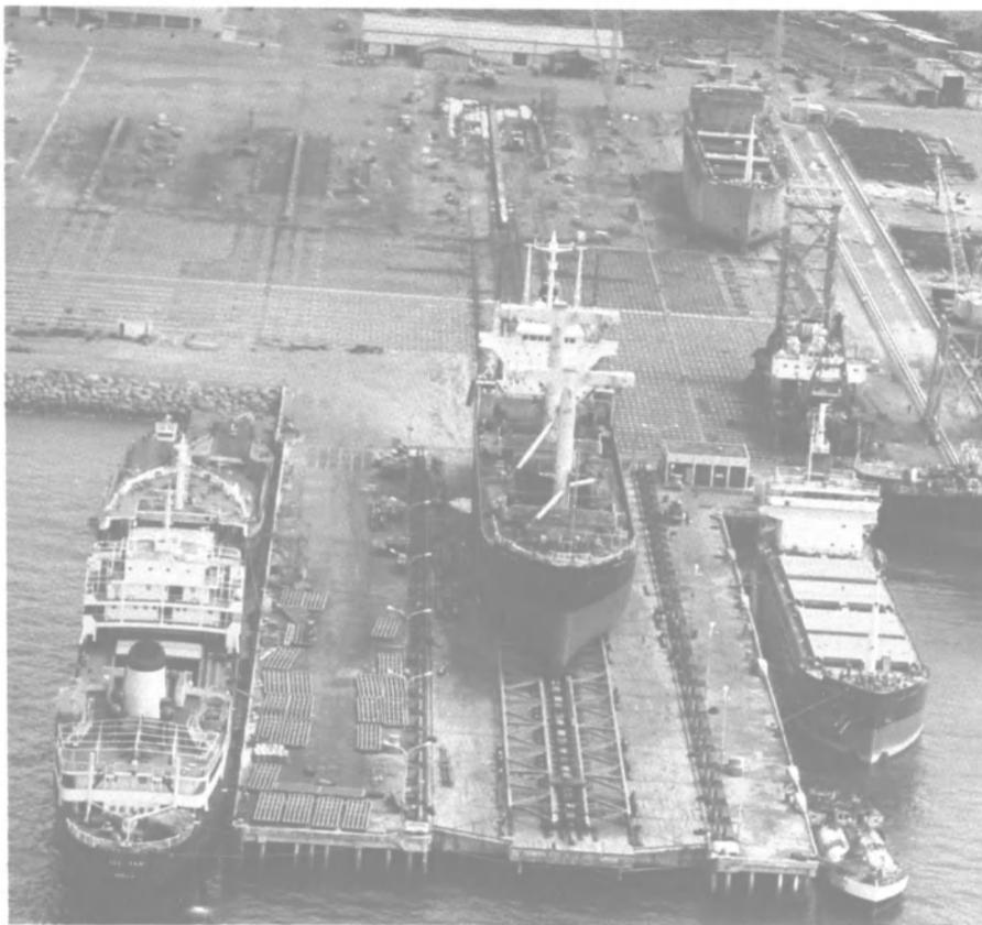
Bogie train positioned under ship on shiplift elevator prior to movement into transfer area on way to repair berth.
