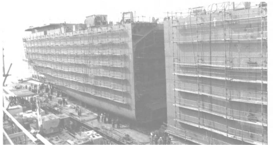
The 3.Maj Shipyard in Yugoslavia built this 34,950-dwt bulk carrier in two parts, a unique technology when the ship is to be launched on an inclined slipway.
