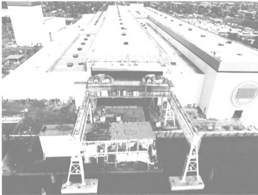
The fabrication facility—11 acres under roof with a 700 ton bridge crane.
