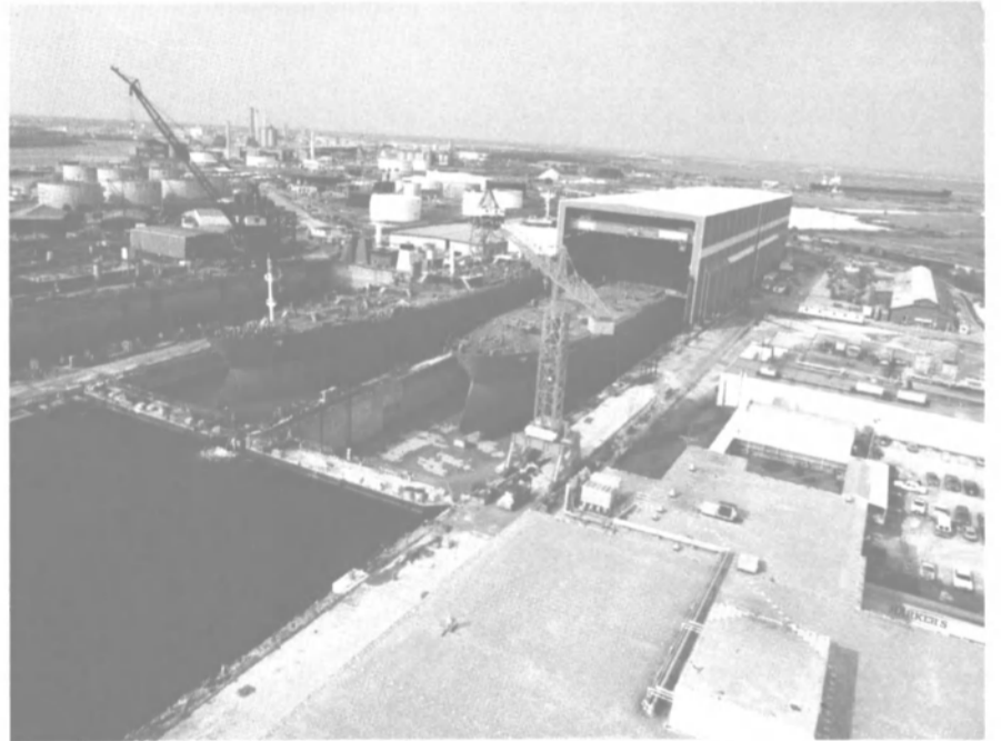
The erection & assembly building—600' x 145' x 115' with three-250 ton bridge cranes—spans 350' of Dry Dock No. 4.
