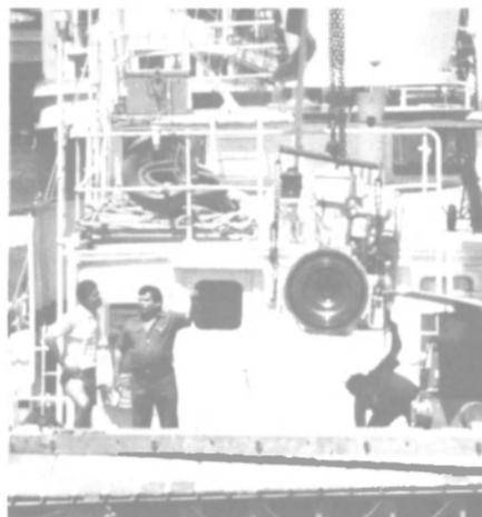
A 500-bhp Cummins KTA19-M marine diesel, one of two that will repower the research vessel Calypso, is lowered into engine compartment at Merrill Stevens Shipyard.
