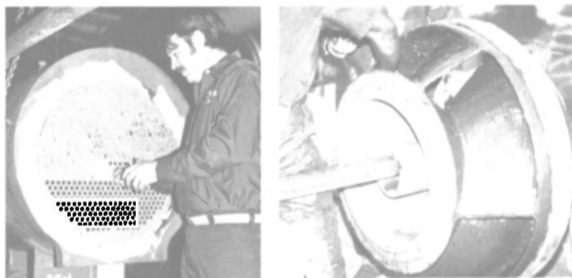
REPAIRING WORN, HEAT EXCHANGER
