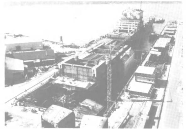
Bay Shipbuilding's 1,158-foot graving dock, where hulls for the three containerships were constructed.
