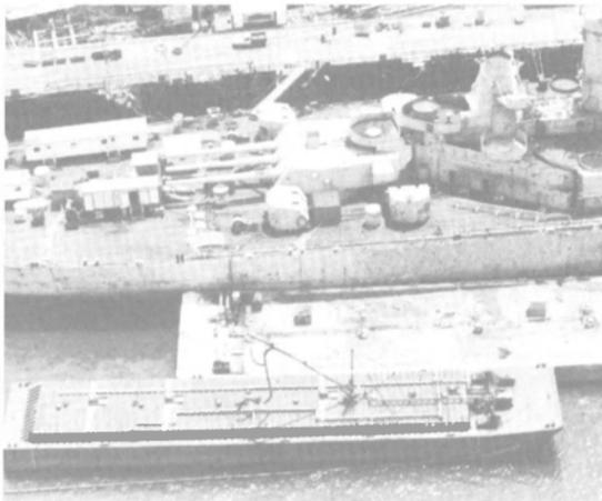
A Koch-Ellis bunkering barge (foreground) is in position to handle MARPOL oily waste water removal from the battleship USS Iowa, which is being renovated at a shipyard near New Orleans.
