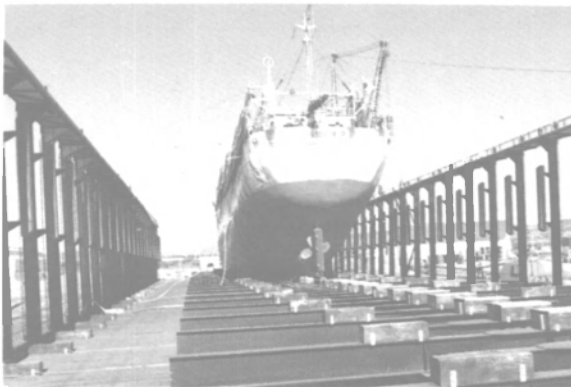
The Crandall Dry Dock-designed 4,000-ton railway in Punta Arenas, Chile, showing vessel on transfer car.
