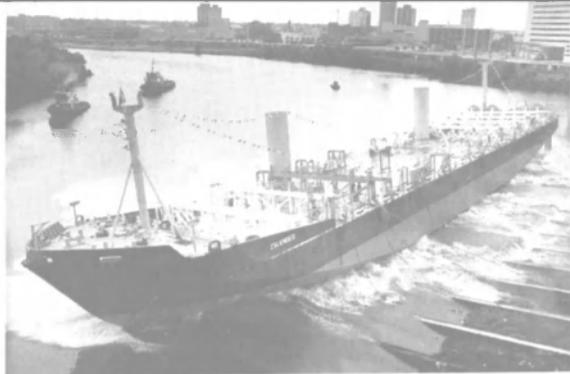
**MAKING WAVES**—Matson Navigation Company's new 387-foot container barge *Islander* slides in to the Neches River from the launching ways at Bethlehem Steel Corporation's Beaumont, Texas, shipyard. The *Islander* has a 316-container capacity and will be used in Matson's mid-Pacific service.
