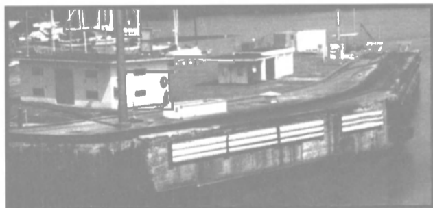
SOLIDUR fender facing in canal system.
