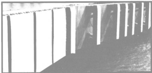
SOLIDUR fender facing on rail ferry terminals.
