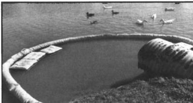
WATERBOOMS and Pillows deployed around outfalls.
