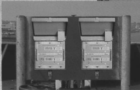
ONDECK DISPLAY, CARGO GAUGING AND OVERFILL PROJECTION, PORT AND STARBOARD TANKS.
