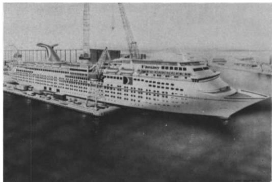
40 miles of 2 Part Life Calk are being installed on Carnival Cruise Lines' newest ship FANTASY at Wartsila Marine, Helsinki, Finland.
