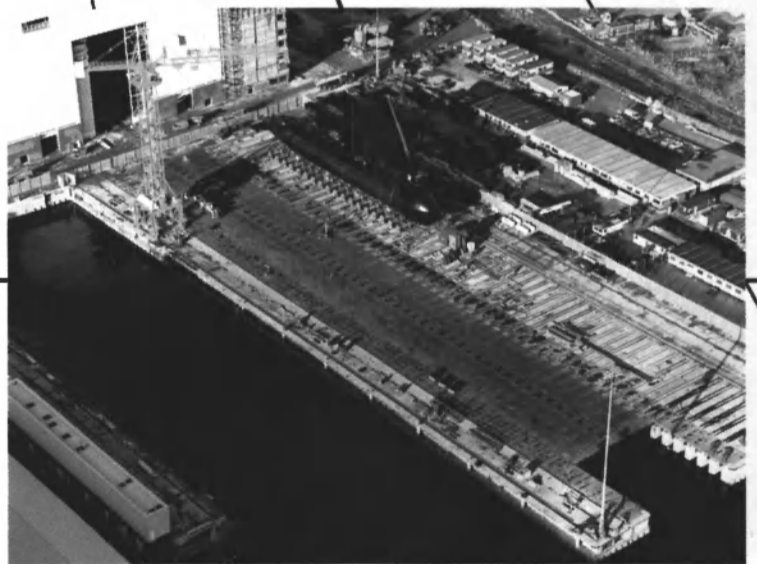
Vickers Shipbuilding and Engineering Works Ltd. Barrow-In-Furness, United Kingdom. Maximum Shiplifting Capacity - 25,000 Tons. Latitude 54.07N Longitude 3.14W.
