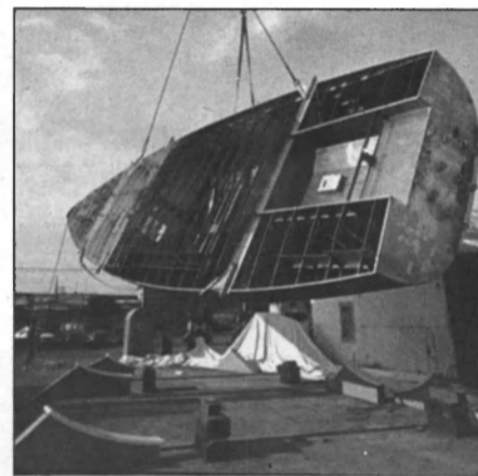
Quiet Cove's 60-foot, solo-racing yacht under construction.
