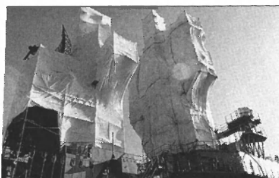
Closures of polyethylene fire-retardant heat shrink wrap capture particulates and reduce cleanup requirements at Southwest Marine, Inc., San Diego.
