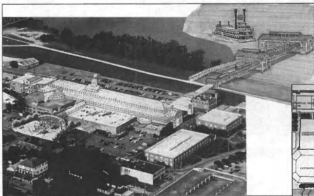
The Phase I renovation of Catfish Town includes a glass enclosure for the existing Catfish Town courtyard. Passengers will use an elevated walkway past Louie's on the Levee onto a walkway with moving sidewalks to load the Catfish Queen .
