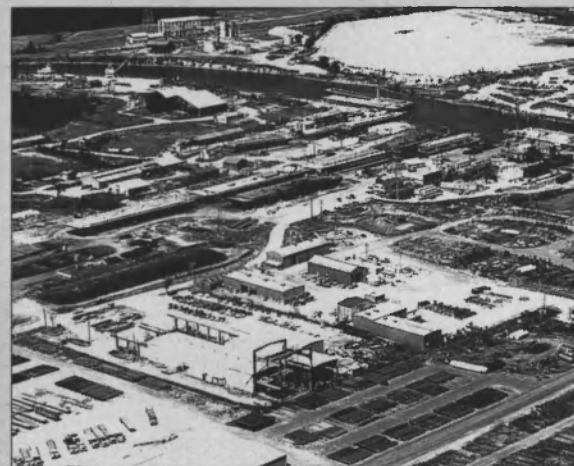
Trinity's new Houston yard, formerly Plotzer Shipyard, Inc.
