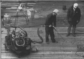
Custom BoatLIFE products and machinery are designed to ease deck sealing and maintenance operations.
