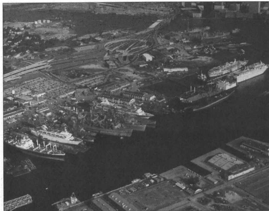
Norshipco's Berkley Plant is the hub of its operation, and home of the Titan, a 950-ft.-long floating steel drydock.
