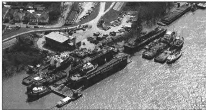
Algiers Iron Works Algiers, Louisiana
