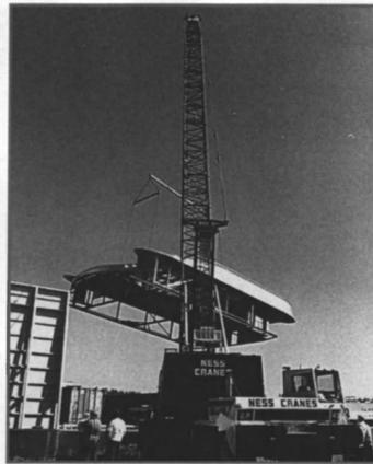
The thin plate and complicated structure of the *Navatek II* superstructure illustrates the type of plates and shapes prepared by Northwest Plasma Cutting. Northwest Plasma Cutting's M.G. cutting machine is located in a high bay building with overhead cranes and truck-wide doors to facilitate handling of raw and finished plates and shapes.
