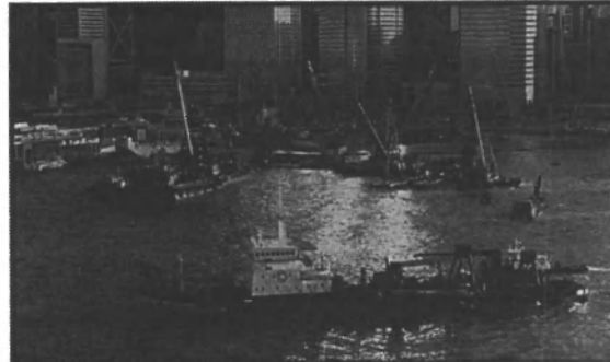
BELOW: Work on Central Reclamation Phase I is shown underway.
