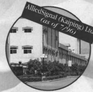
Guangdong, China (Technical Center/ Manufacturing)
