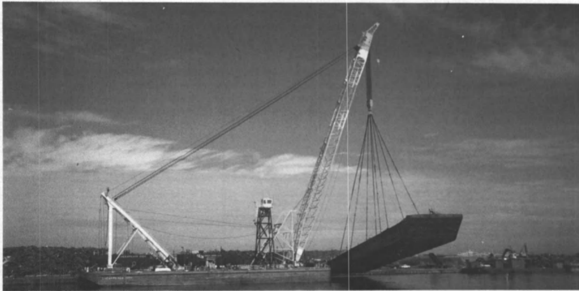
Derrick Barge CHESAPEAKE 1000
