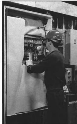
Electro-Shield insulated rubber shielding conforms to both O.S.H.A. 1910.335 Safety Related Work Practices and ASTM-D-178 Specifications for Type II Matting.
