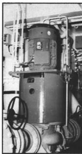
The range features 15 models of the Dolphin centrifugal pumps, which address 75 percent of ship-board pumping duties. They include main engine cooling, auxiliary cooling water circuits, bilge systems, ballast systems and general service.
