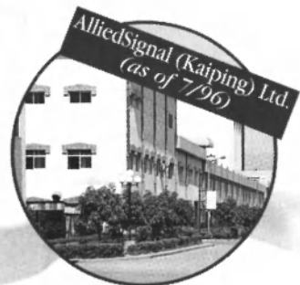
Guangdong, China (Technical Center/ Manufacturing)
