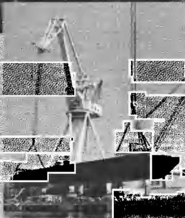
Spar caisson weldout of the FPS Neptune "next-generation" offshore production platform. Ingalls fitted and joined two massive, 72-foot diameter caissons together — a historical first — to form the 705-foot-long Spar hull, and completed the installation of spiral hull strakes to stabilize the structure against ocean currents.
