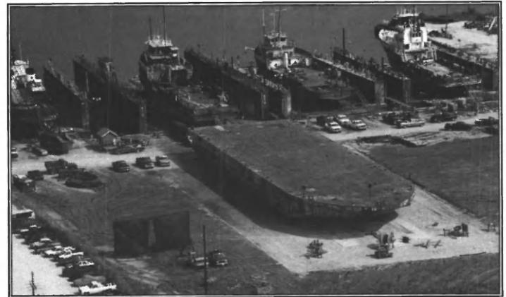
Located on the Gulf Intracoastal Waterway at mile marker 36, Bollinger's Larose Division offers repair of both steel and aluminum vessels and works around the clock to satisfy the demanding marine industry. Bollinger Larose operates four floating dry docks that can handle vessels up to 6500 tons with 86 ft. between the wings. A newly constructed bow/roll-off transfer system can accommodate up to 3,000 tons of marine equipment.
