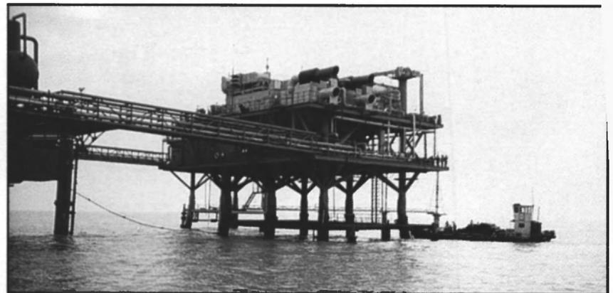
Pictured is an offshore platform with two Heatec waste heat recovery units.
