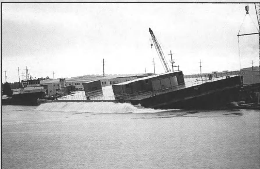
Pictured is the launching of a Bollinger barge derrick.
