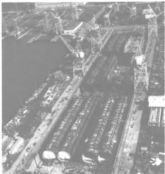
At left: Some of the 15 steel tunnel tube sections under construction at Bethlehem Steel's Baltimore Marine Division. The 300-foot-long sections will be used to build the Interstate 664 tunnel crossing in the Hampton Roads section of Virginia. At right: The USNS Maury (T-AGS-39), the first of two oceanographic survey ships being constructed at Bethlehem Steel-Sparrows Point. She is scheduled for delivery in July.
