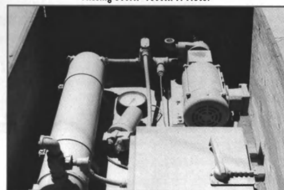
6 Lube Oil Preheaters Mfg: Kim-Hotstart P/N SPOL3P 12044X-FC-1012-SUB Units Include Tuthill Model 2 CEV 6.2GPM Pump Driven By 1 HP 230/460/3'60 | 140RPM Motors
