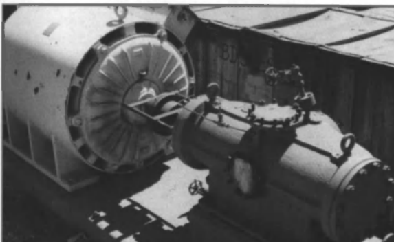
2 Fuel Oil Transfer Pumps Size 8x6 Mfg: DeLaval 700/525/350/250GPM@150psi Horizontal Model A32NX437 Motor: Continental 100/75/50/37.5HP 440/3'60 TEFC
