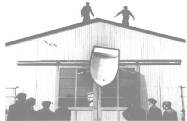
Drop test from the roof of the boatbuilding shed using a plastic rowing boat in 1957.
