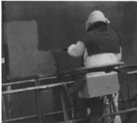
Blasting with METgrain Abrasive
