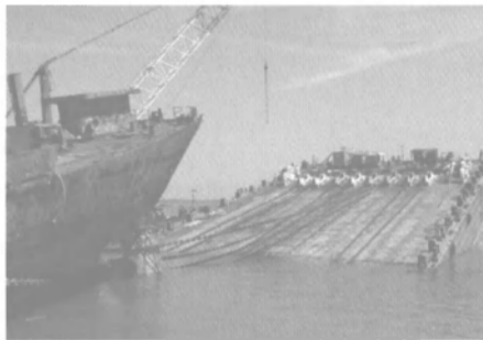
Pulling AN TAI onto the barge
