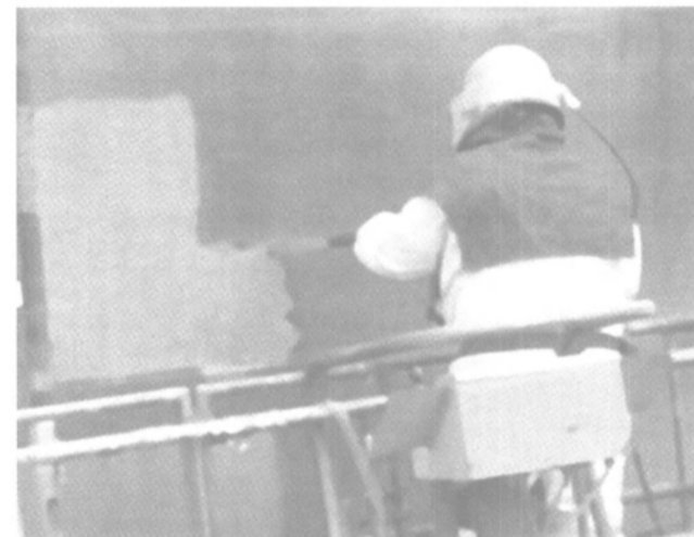
Blasting with METgrit abrasive
