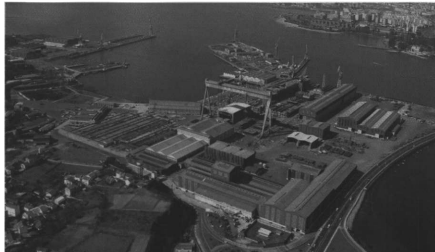
IZAR Fene Shipyard facilities include modern and automatized workshops and paved yard areas, with piers, stores, drydocks, building berths, and mobile and locomotive cranes. An outstanding 800 ton gantry crane spans over both the construction berths and the assembling/pre-erection area and may perform on-board outfitting operations.
