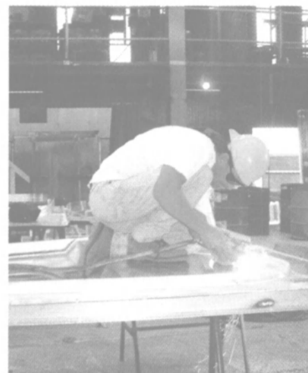
On the job: A welder employed by Blount-Barker Shipbuilding busy at work on the yard's newest innovation — aluminum fast craft construction. (Photo Credit: Regina P. Ciardiello)
