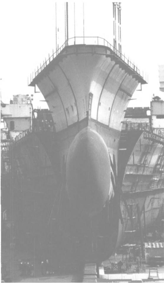
CVN-76 is the first nuclear Aircraft Carrier to sport a bulbous bow, a feature designed to enhance flight operations. The new bow adds 36 feet to the underwater length of the ship.
