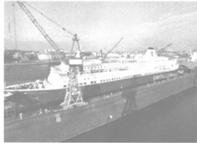
On January 7, 2003, the 664-ft. (202.2-m) passenger/car ferry Prinsesse Ragnhild, which belongs to Norwegian shipowner Color Line, began a 41-day stay at the Blohm+Voss shipyard. The vessel, which has a gt of 35,438, and a breadth of 80 ft. (24.3 m), is to undergo a comprehensive general overhaul of its auxiliary diesel and main starboard engine — and a new coat of paint.
