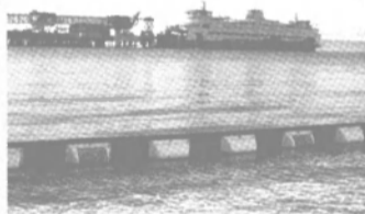
Port Security Barrier
