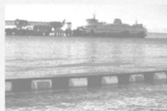
Port Security Barrier
