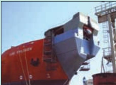
Following 40 days of rebuilding at Remontova yard in Gdansk, Poland, the *Siri Knutsen* was converted into a shuttle tanker. The company's KVOC tank system concept installed during the rebuilding.
