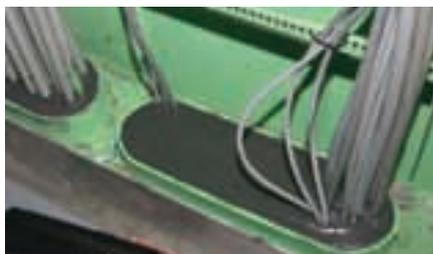
protective sleeves that are split lengthwise and are simply placed around the cables. Once the cables to be ducted have been packed in this way, the remaining space is filled up with empty filler sleeves. Lastly, the penetration is closed off with a 2 cm thick layer of fire resistant, water repellent and gas tight FIWA compound. In order to be able to add extra cables at a later date, it is only necessary to cut away the FIWA com-
