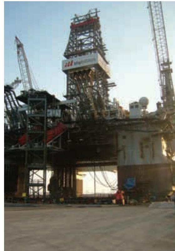
Work on Development Driller 1 included reinforcement of areas in the lower pontoons, located above the four thruster rooms on board the semi-submersible drilling rig.
