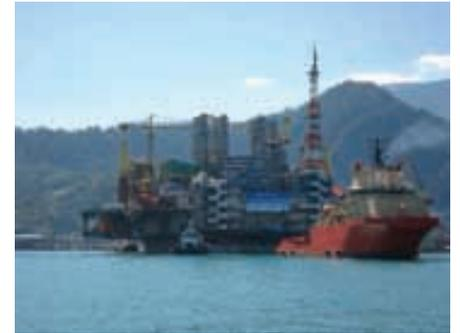
Towing the P-52 deck box to mate with the lower hull.
