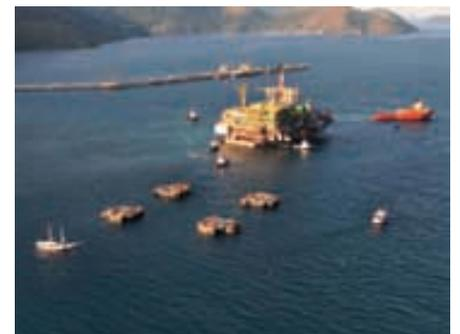
Positioning the deck box to meet the lower hull.
