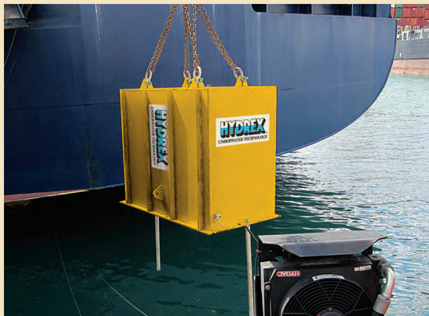
Hydrex designed a tailor-made cofferdam for a RoRo propeller fix.
