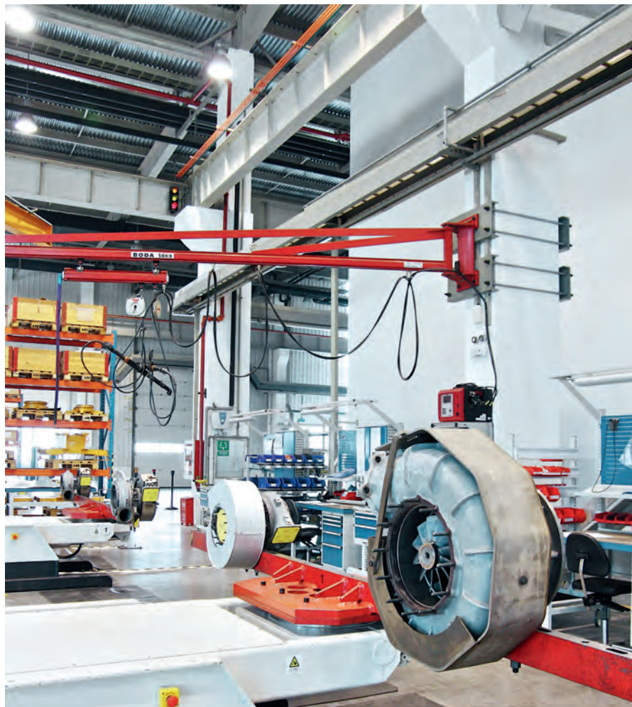
The factory of ABB Jiangjin Turbo Systems Co., Ltd. is one of the most modern turbocharger facilities in the World.
