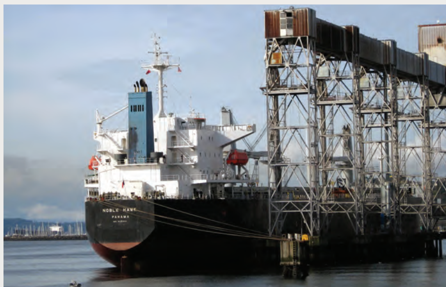
Responsibility for providing emergency back-up power for air filtration at a grain loading facility is too important to wait until the grid fails before considering options.
