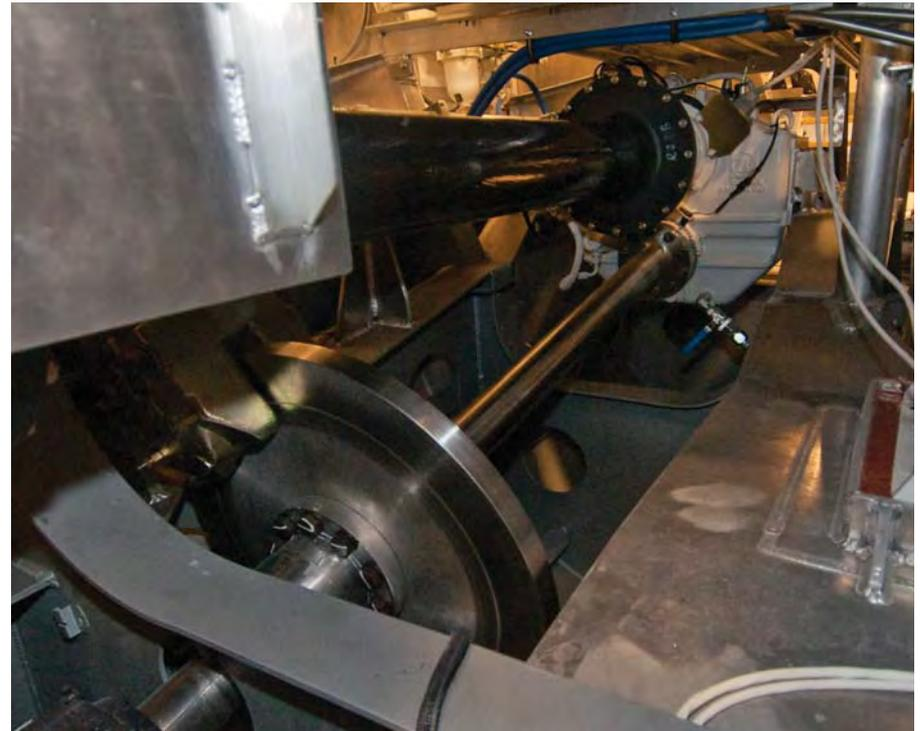
**ZF Marine supplied the complete propulsion system, apart from the engines, including this ZF550 V-drive gear and shaft brake for the smaller C18 engine.**
