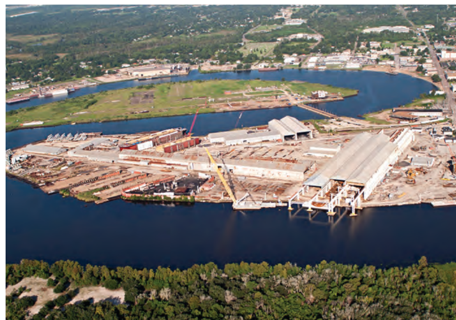
Signal International Texas Yard.
